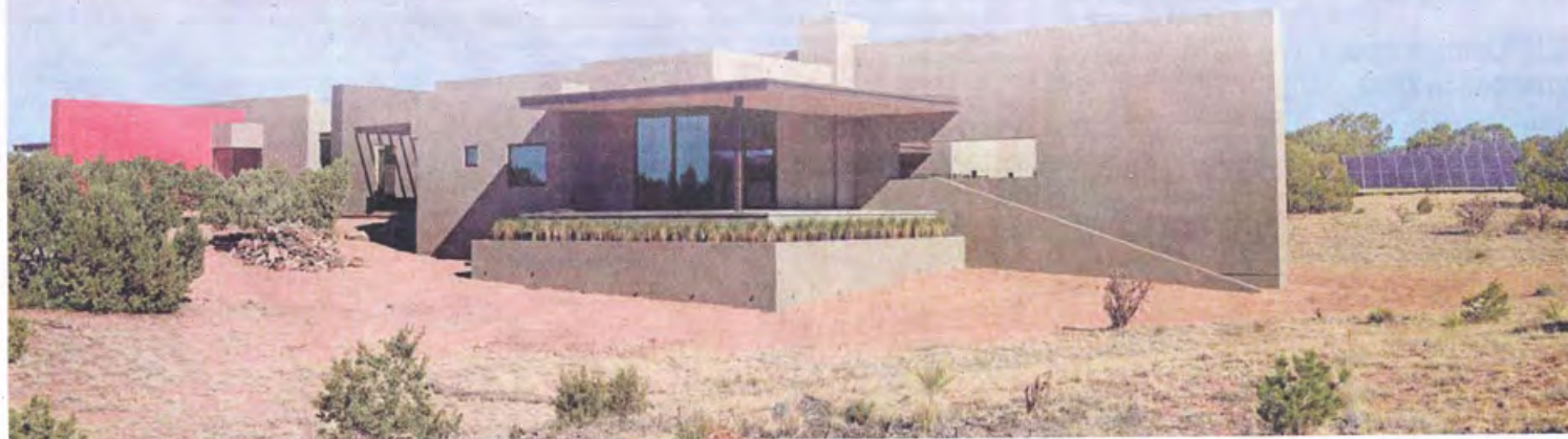
After two years of construction, an 8,000-square-foot home nears completion at the Galisteo Basin Preserve. The home, which is owned by a couple from Nashville, Tenn., features a man-made waterfall, half a dozen bathrooms, two kitchens and a room designed to house the couple's cats. PHOTOS BY CLYDE MUELLER/THE NEW MEXICAN
